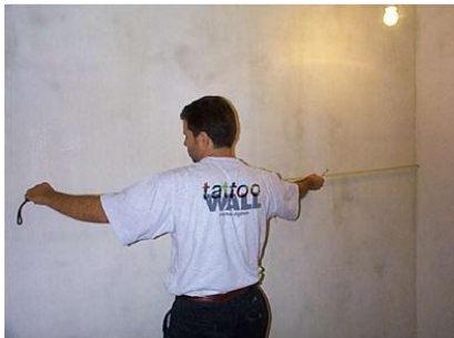
8. Mark the centre horizontal line of the surface that will be decorated. Take the first Tattoowall™ print.
