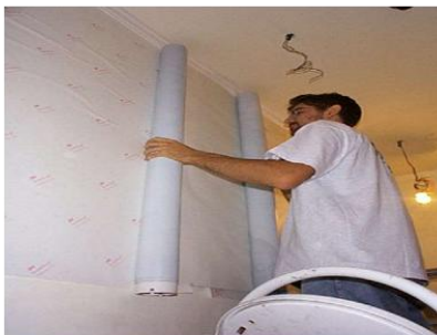
12. This will help to position the Tattoowall™ without it adhering to the P2M before centering has taken place.
