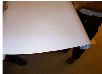
10. The first print will be recognizable by a mark that indicates the horizontal centre. This mark will be positioned to correspond with the mark on the wall.
