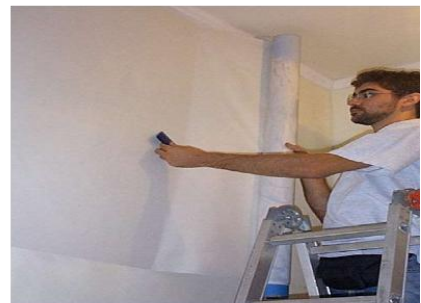
13. Once the sheet has been correctly centered, begin to smooth it out, starting from the center towards the edges, using a “fish bone” motion. Once this operation is complete it is important to repeat the center mark of the wall on the Tattoowall™.
